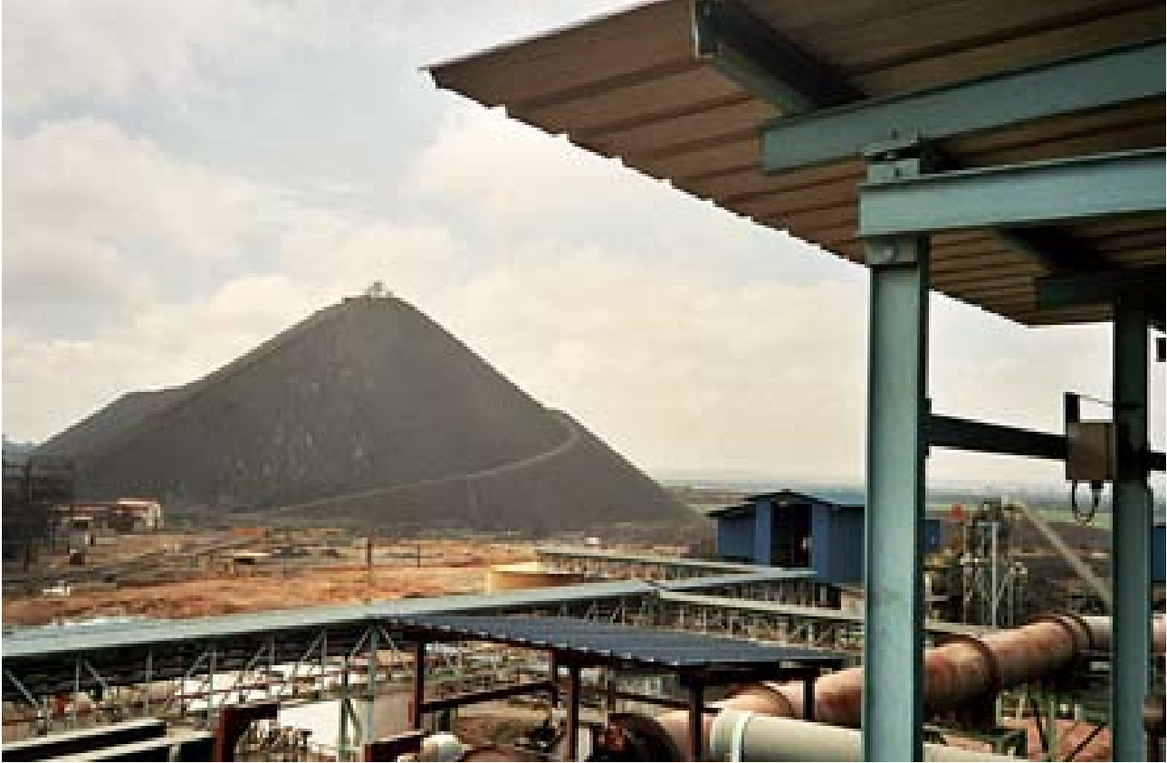
The GTL/STL plant in Lubumbashi (Photo IPIS)
